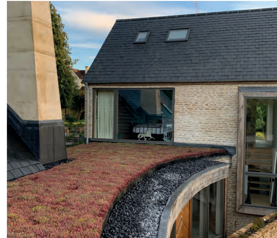
Green or brown roofs can be low maintenance and provide a wildlife habitat, reduce surface run-off, provide shade, remove heat from the air, and reduce temperatures of the roof surface, St. Mary Street
