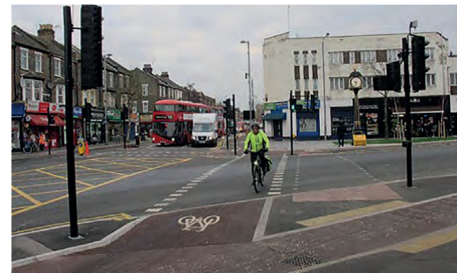
Signalised cycle crossing gives priority to cyclists over motorised traffic at road junctions, Waltham Forest
