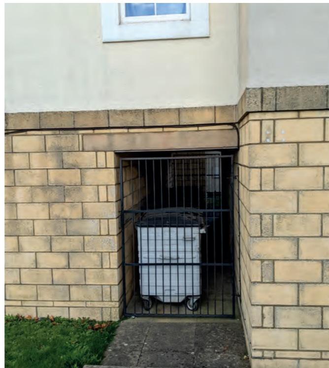
Space for commercial wheelie bin storage can be integrated into the building design, Queens Square
