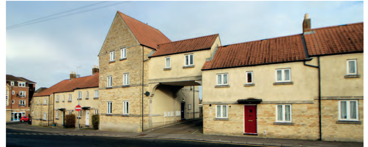
Development which contains rear courtyard parking is successful in areas with strong 'urban' character. Benefits include removal of vehicles from the street and creation of a strong building line, Bakehouse Close
