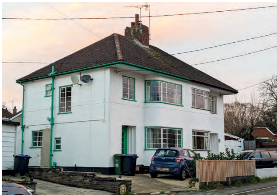
Art-Deco style Inter-War houses are attractive where original window features have been retained, Deansway
