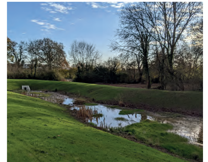
SuDS incorporated into green infrastructure have recreational, ecological and flood alleviation benefits, North Chippenham
